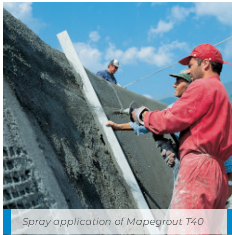
Finishing of Mapegrout T40
