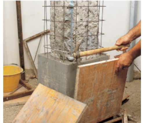
Removing wooden formwork
