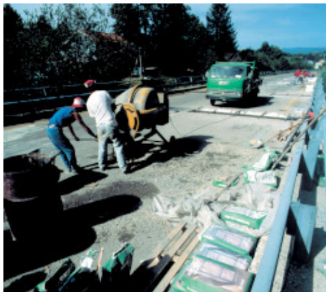
Reforming road joints
