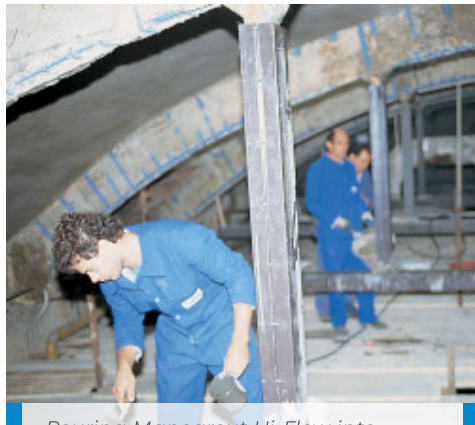
Pouring Mapegrout Hi-Flow into metal formwork
