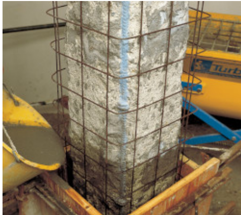
Pouring into a formwork
